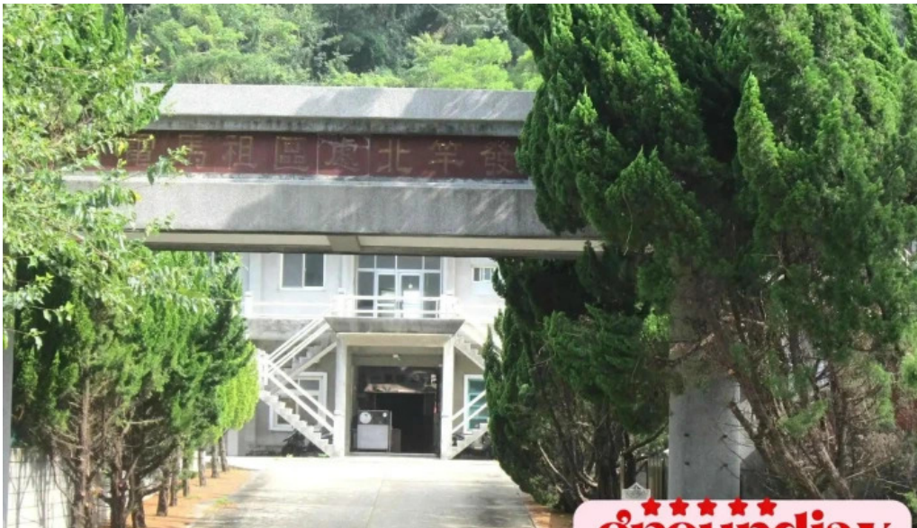
Taiwan power company Quan Bu
