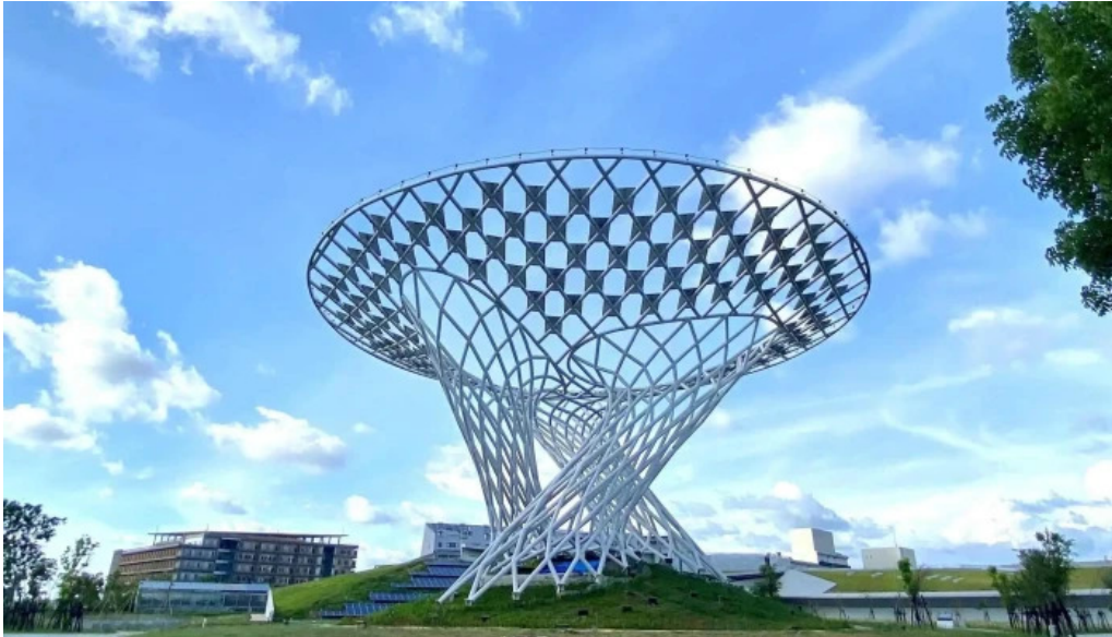
Industrial technology research institute shalun ??
