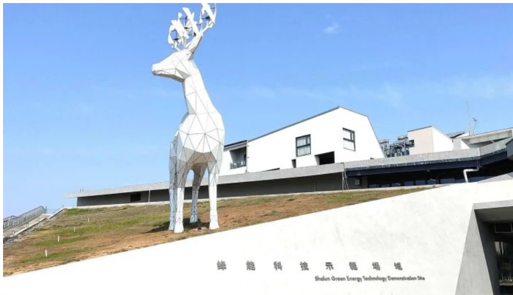
Industrial technology research institute shalun ????
